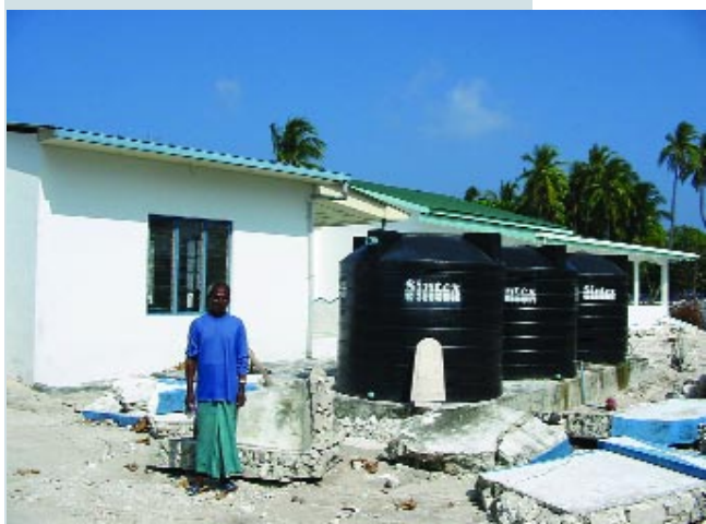
Water storage tanks in the Maldives.
