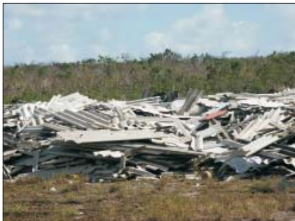
Source: Asbestos containing roof debris after cyclone, Fiji
