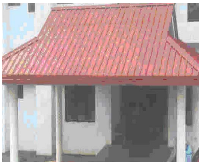
Roofing Substitute for Asbestos
