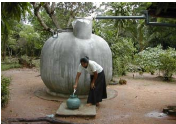
Rain Water Harvesting helps get safe drinking water at door step.
