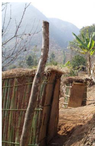
Currently there are over 120 ecosan toilets. Some are made using split-bamboo walls
